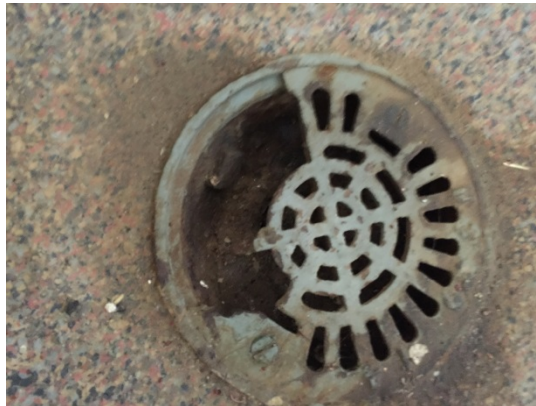
Photograph 2: Interior floor drain in the restroom identified in Photograph #1.
