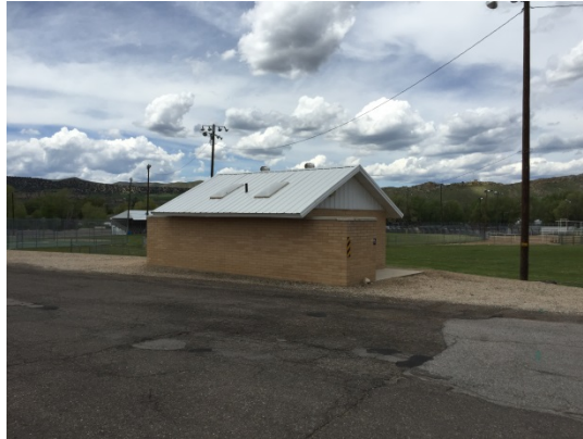
Photograph 25: Brick restrooms located near the south central portion of the property, south of the southeastern baseball diamond.
