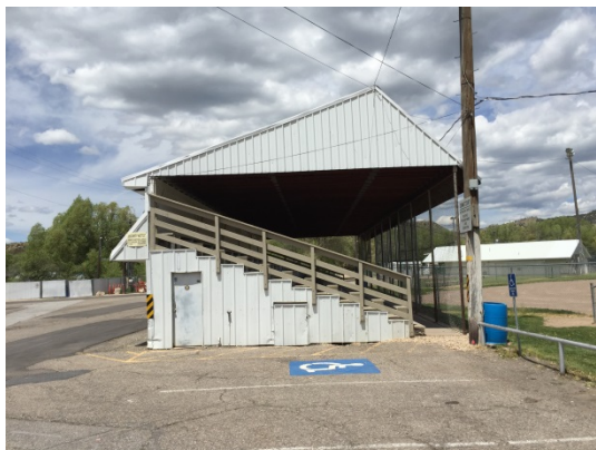
Photograph 18: Grandstands located near the western central portion of the property, adjacent to the parking lot.
