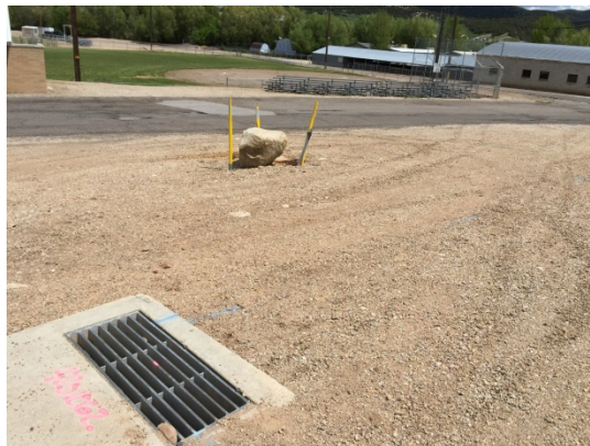
Photograph 12: Concrete catch basin located southwest of the artesian well.
