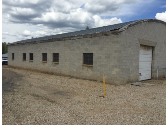
Photograph 22: Livestock building located near the southeastern corner of the property, adjacent to the eastern property boundary.
