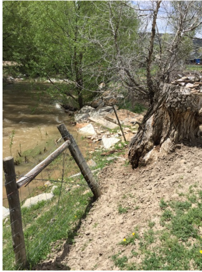
Photograph 13: Concrete debris located adjacent to Chalk Creek.
