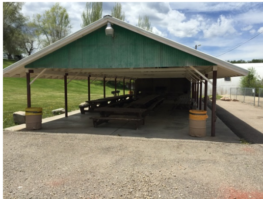
Photograph 14: Covered picnic area located south of the playground area, near the western property boundary.
